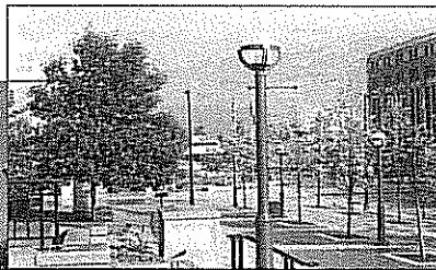
MLK, Jr. Blvd Improvements
